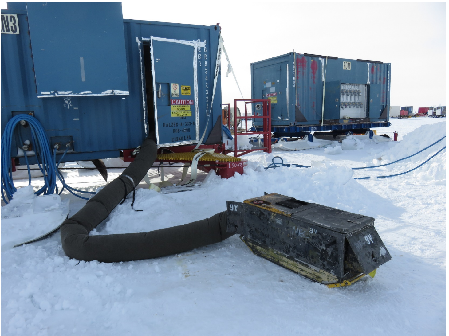
Preheating Generator 3 before testing
