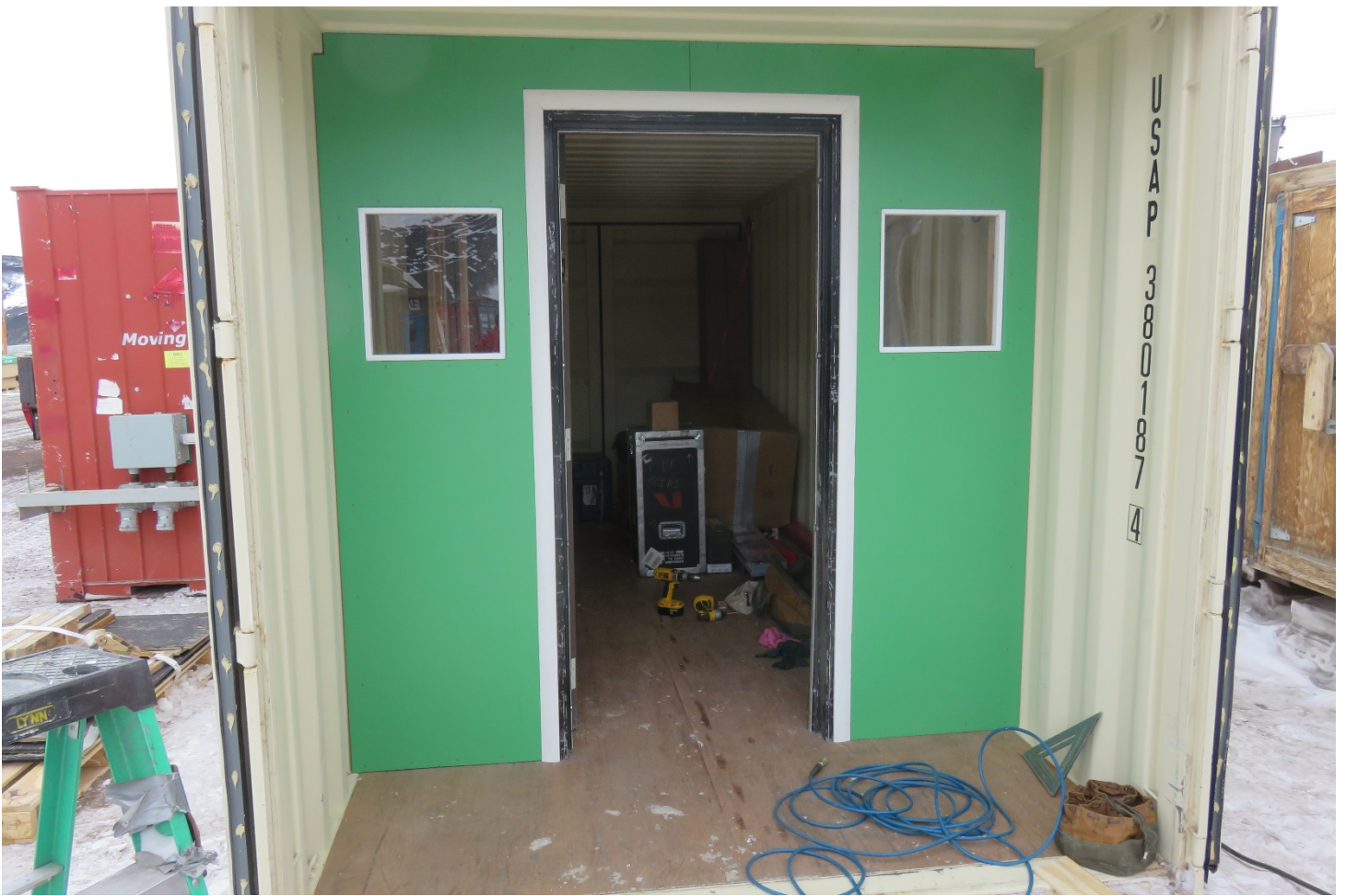
C&C, further along and some very good workmanship, Photo by Dennis Duling
