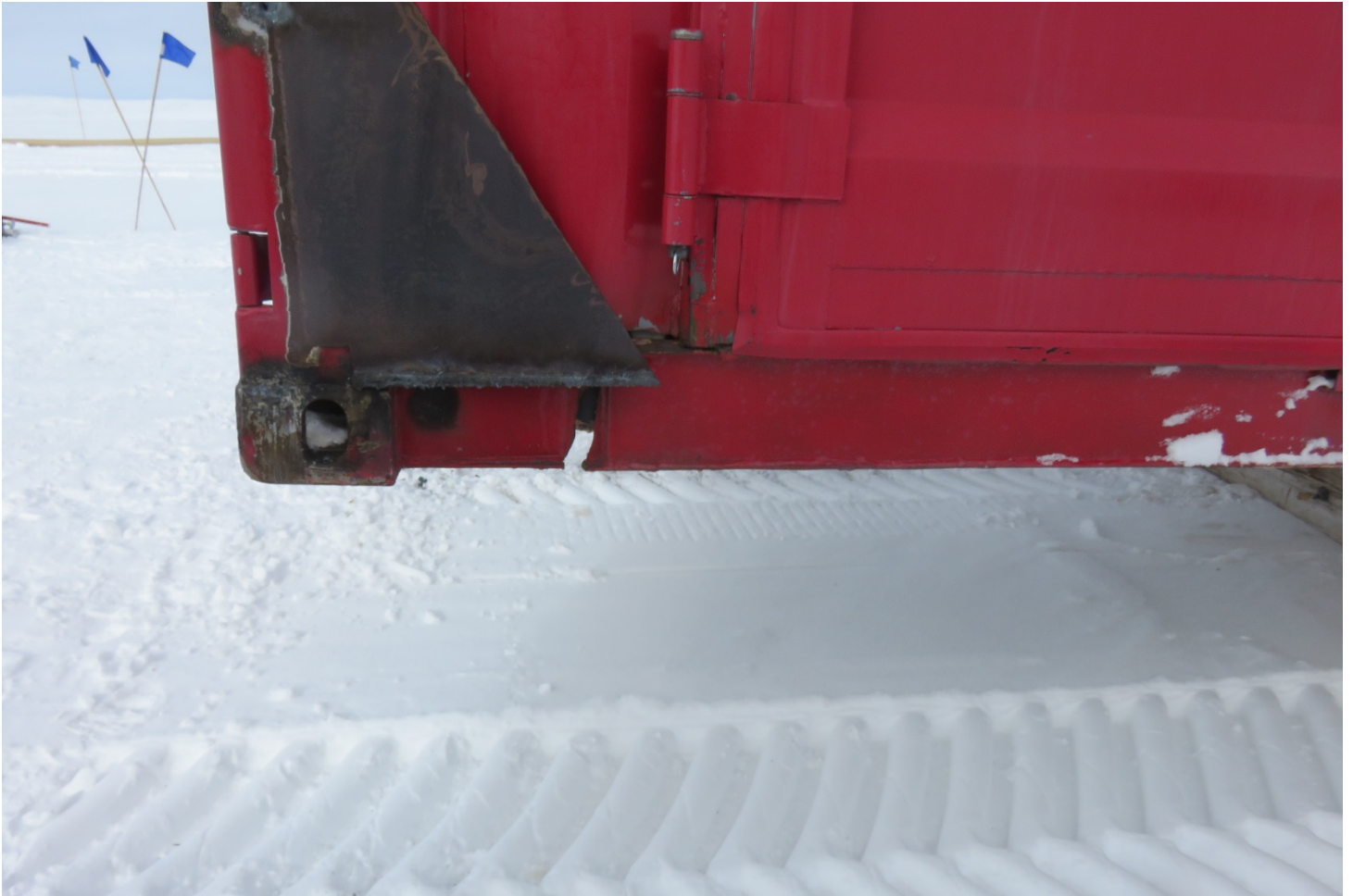
HPU-1 damage, main frame broken free from the structural corner and container door frame. Photo by Dennis Duling
